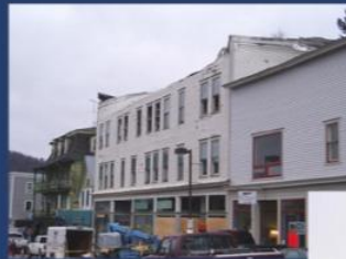
Bemis Block - 73 South Main Street
