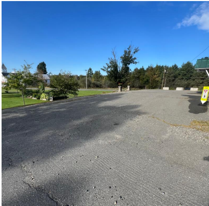
82 CRAFTSBURY ROAD – UPPER-LEVEL PARKING
