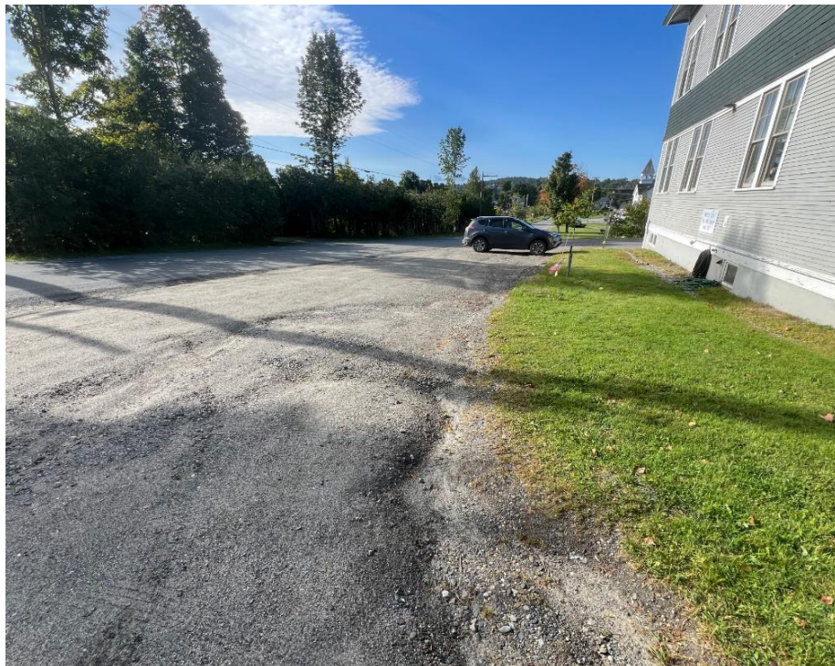
82 CRAFTSBURY ROAD – UPPER-LEVEL PARKING
