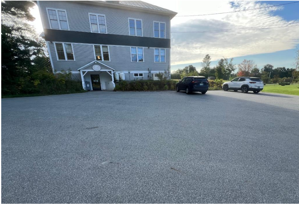
82 CRAFTSBURY ROAD – UPPER-LEVEL PARKING
