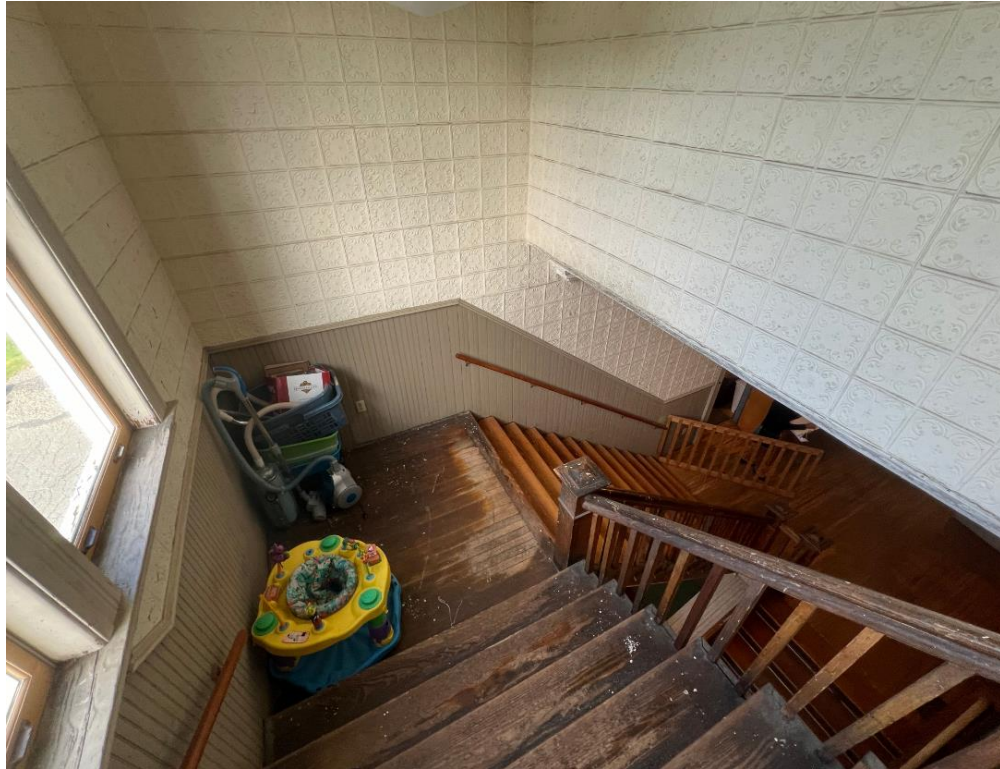
82 CRAFTSBURY ROAD – SECOND FLOOR STAIRWAY
