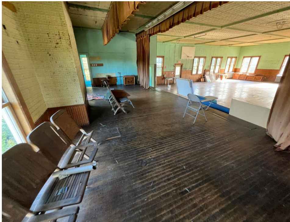
82 CRAFTSBURY ROAD – SECOND FLOOR STAGE
