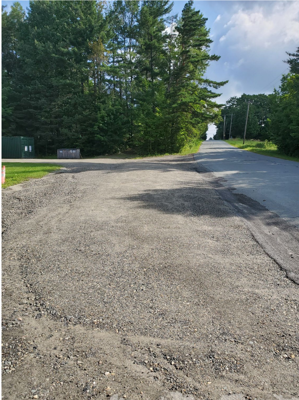
Photo # 9 Driveway entrance along Lauredon Ave.
