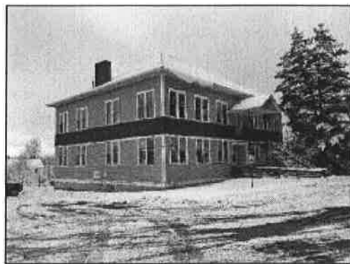
Exterior – NE corner
