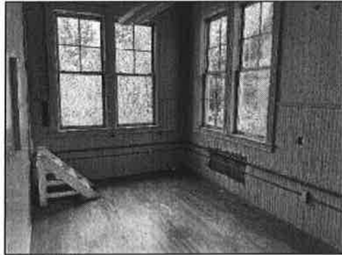
Interior, 2 nd floor – room
