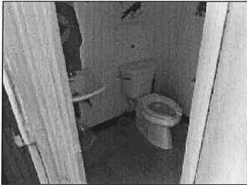
Interior, 1 st Floor – 2-fixture bath
