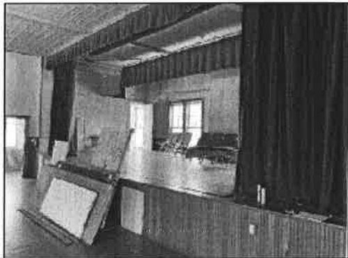
Interior, 2 nd floor – stage
