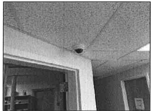
Interior, Lower Level - security
