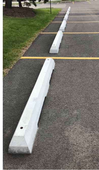
Above: Concrete wheelstops placed at least two feet from the curb would be a suitable permanent solution.
