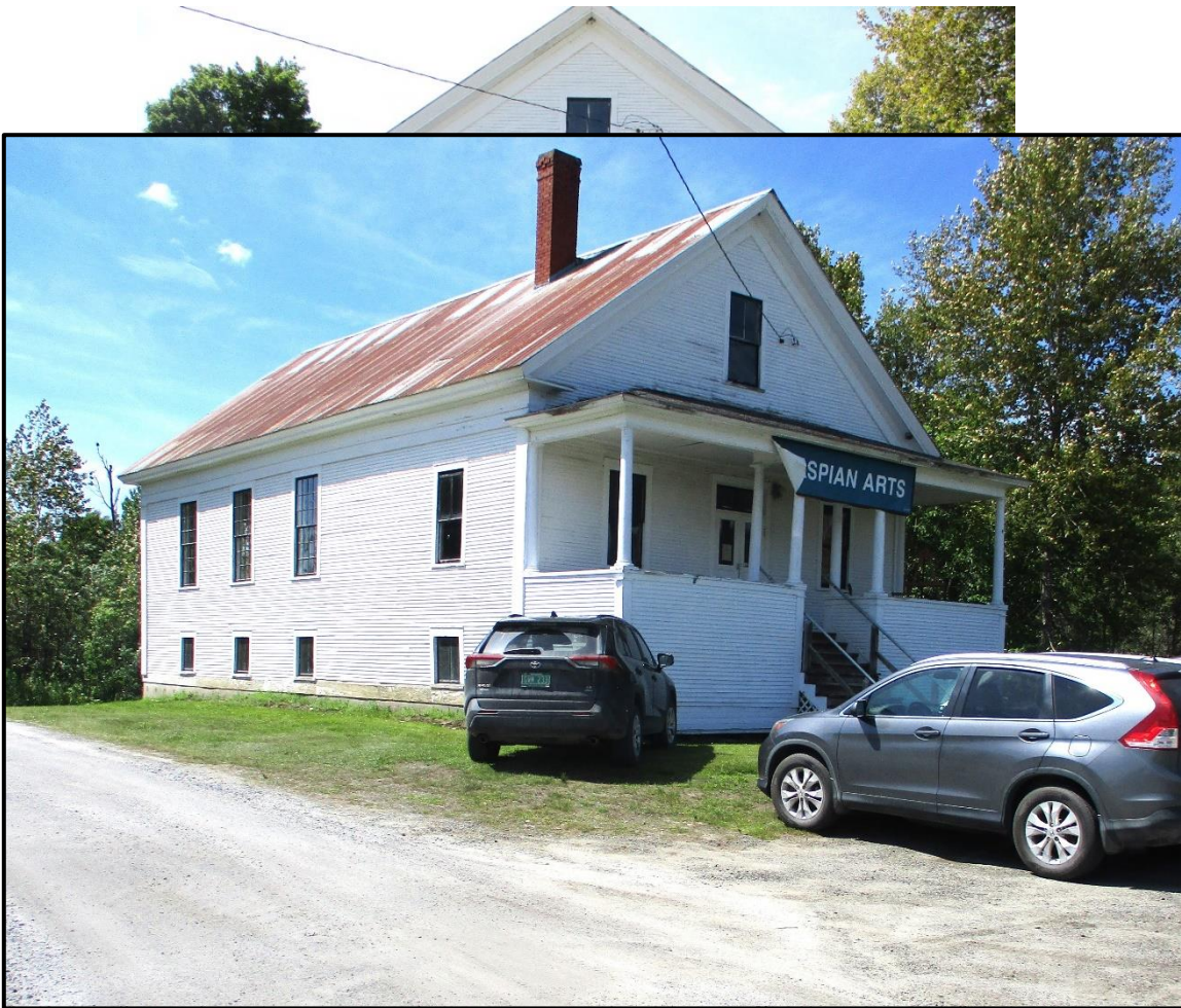
The easterly front of the building and the covered entry porch.
