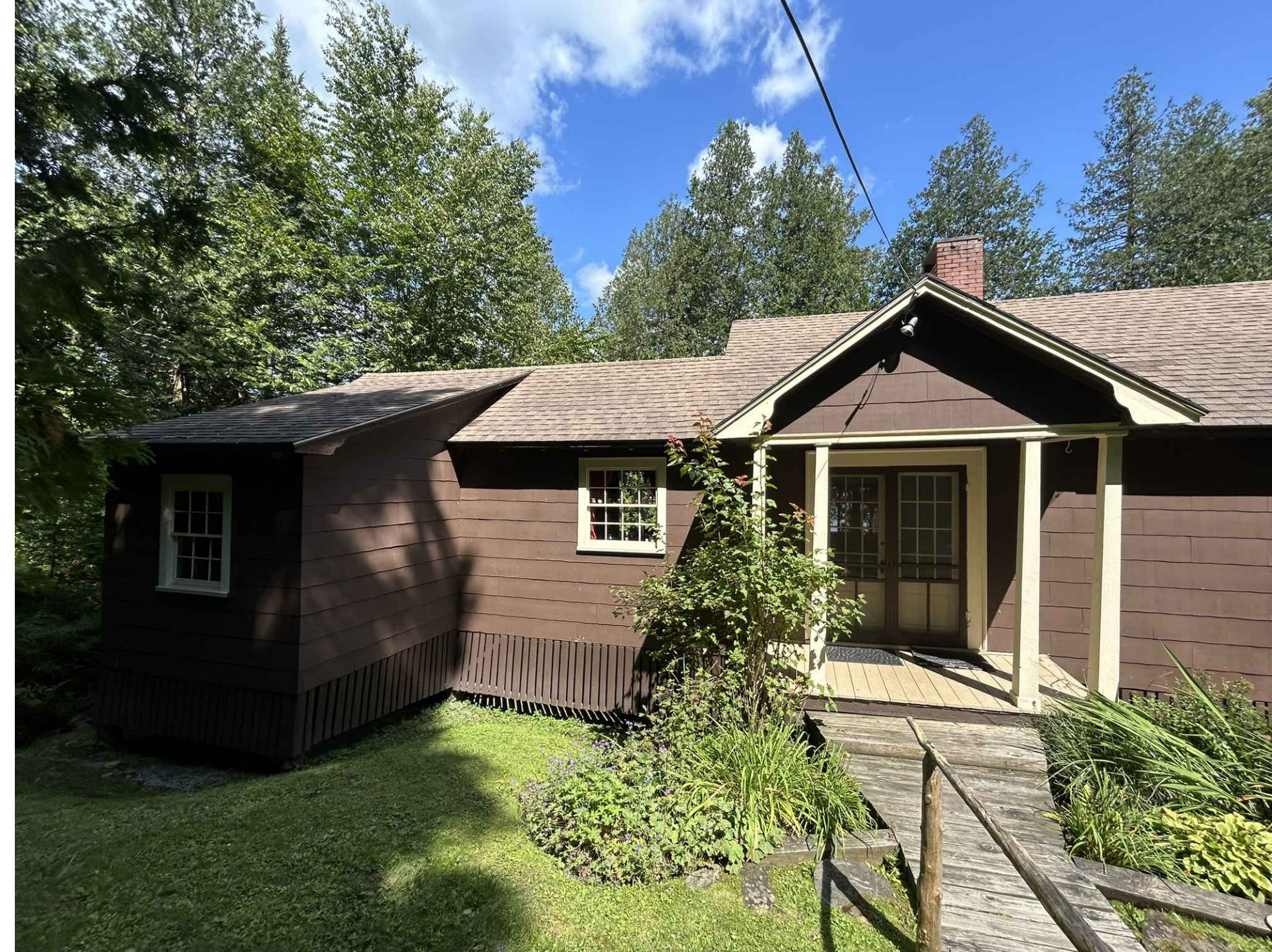
PHOTO OF EXISTING HOUSE ENTRY PORCH & NORTHWEST HOUSE CORNER (LOOKING NORTHEAST)
